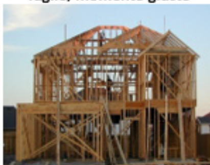
Posa in opera
